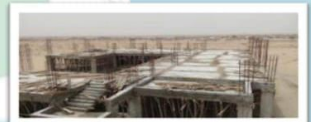
Academic Block I (under construction):- 36.53 %
