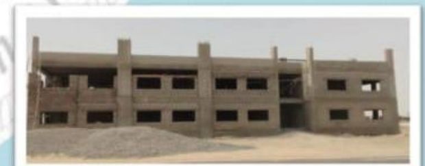
Academic Block II (under construction):-61.03 %
