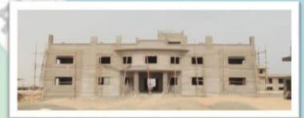
Admin Block (under construction):-71.50 %
